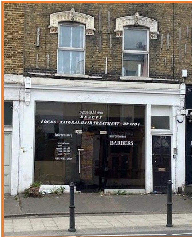
Ground Floor Shop, 57 Lavender Hill, London SW11 5QN
